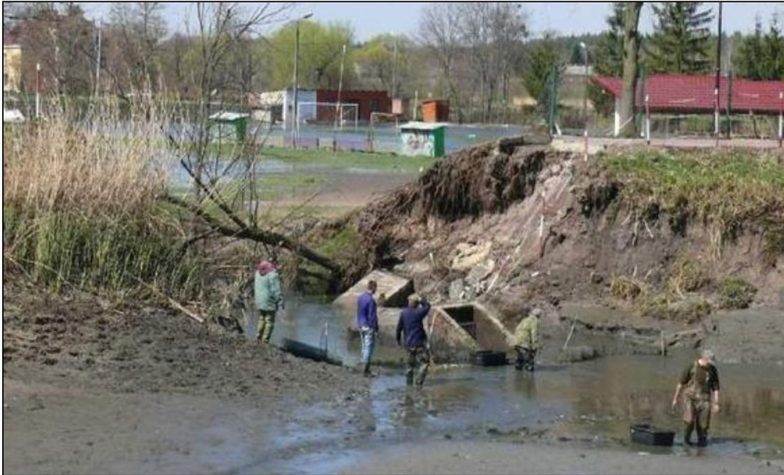
Figure 2: Burst dam on a fish pond in Zaklików in 2012 (<http://wiadomosci.onet.pl/Kielce>).
