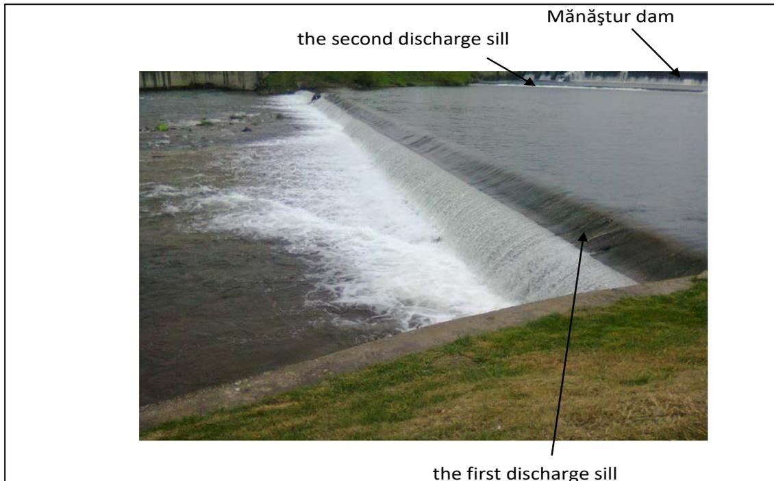
Figure 3: The first discharge sill downstream of Mănăștur dam.
