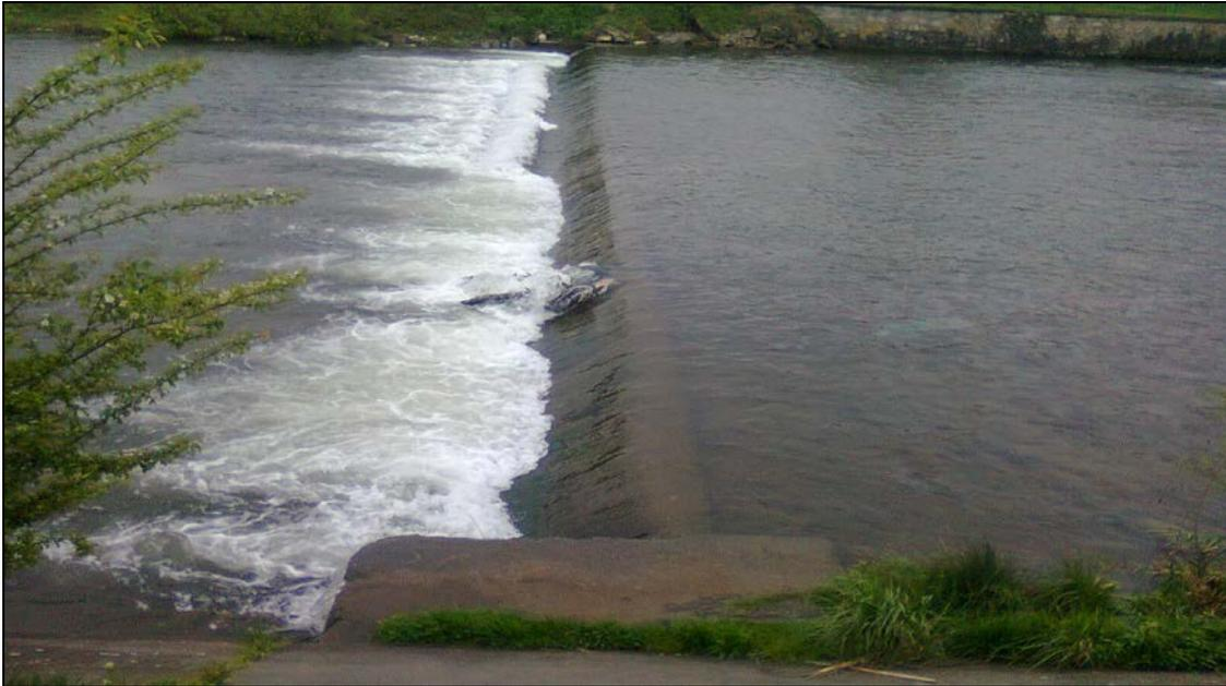
Figure 15: The second discharge sill located near Mănăştur dam.
