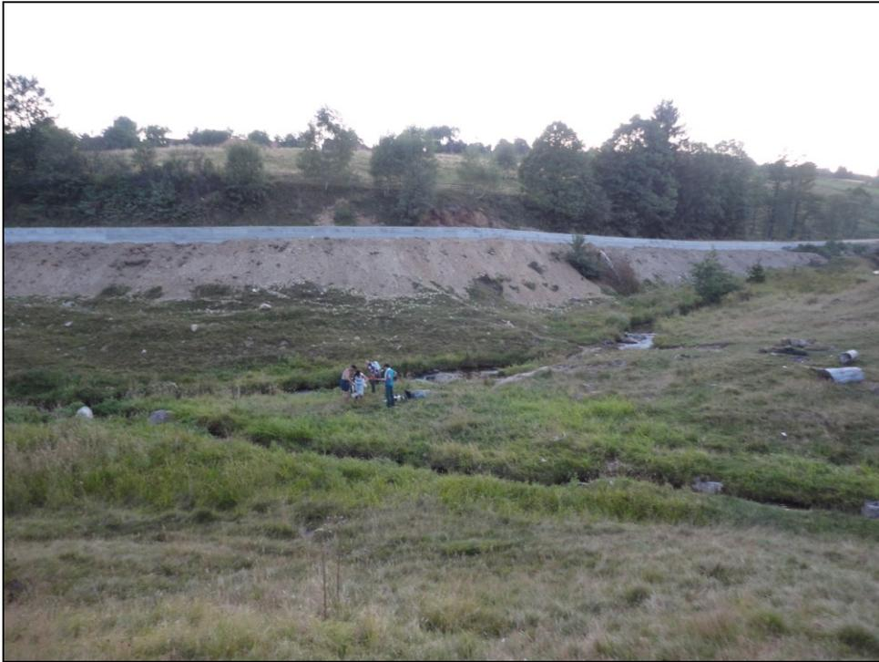
Figure 5: Loose slopes, on the roadside of Brebu-Slatina Timiș near the Lung Stream, increase sedimentation and habitats degradation impact on salmonids.
