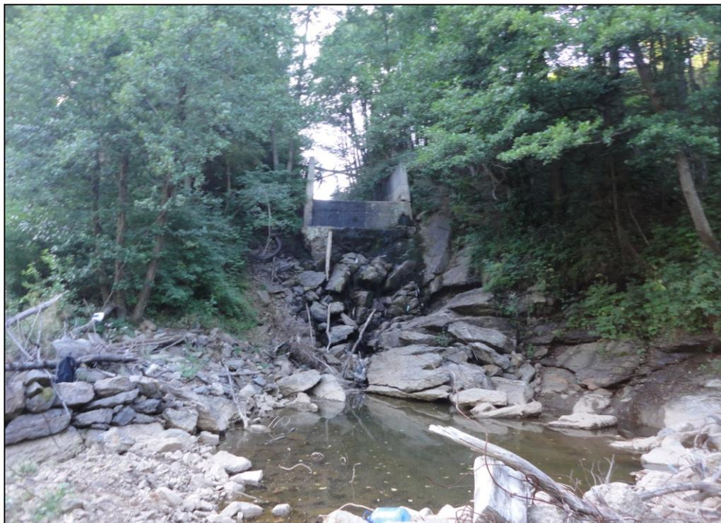
Figure 9: The lotic discontinuum due to Three Waters Dam - the overflow spilway of the dam.
