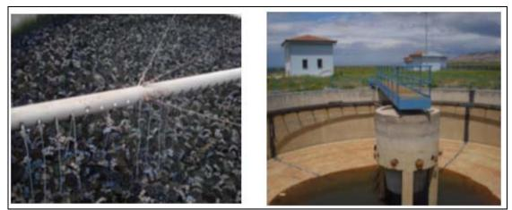
Trickling filter tankSedimentation tankFigure 6: Develi Wastewater Treatment Plant (photo Ferit Yuksel, 2008).
