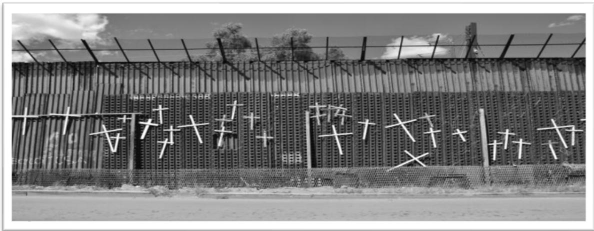
Figure 4. Section Built from a Steel Landing Mat. The Crosses Commemorate Those Who Died Attempting to Cross the Border 4
